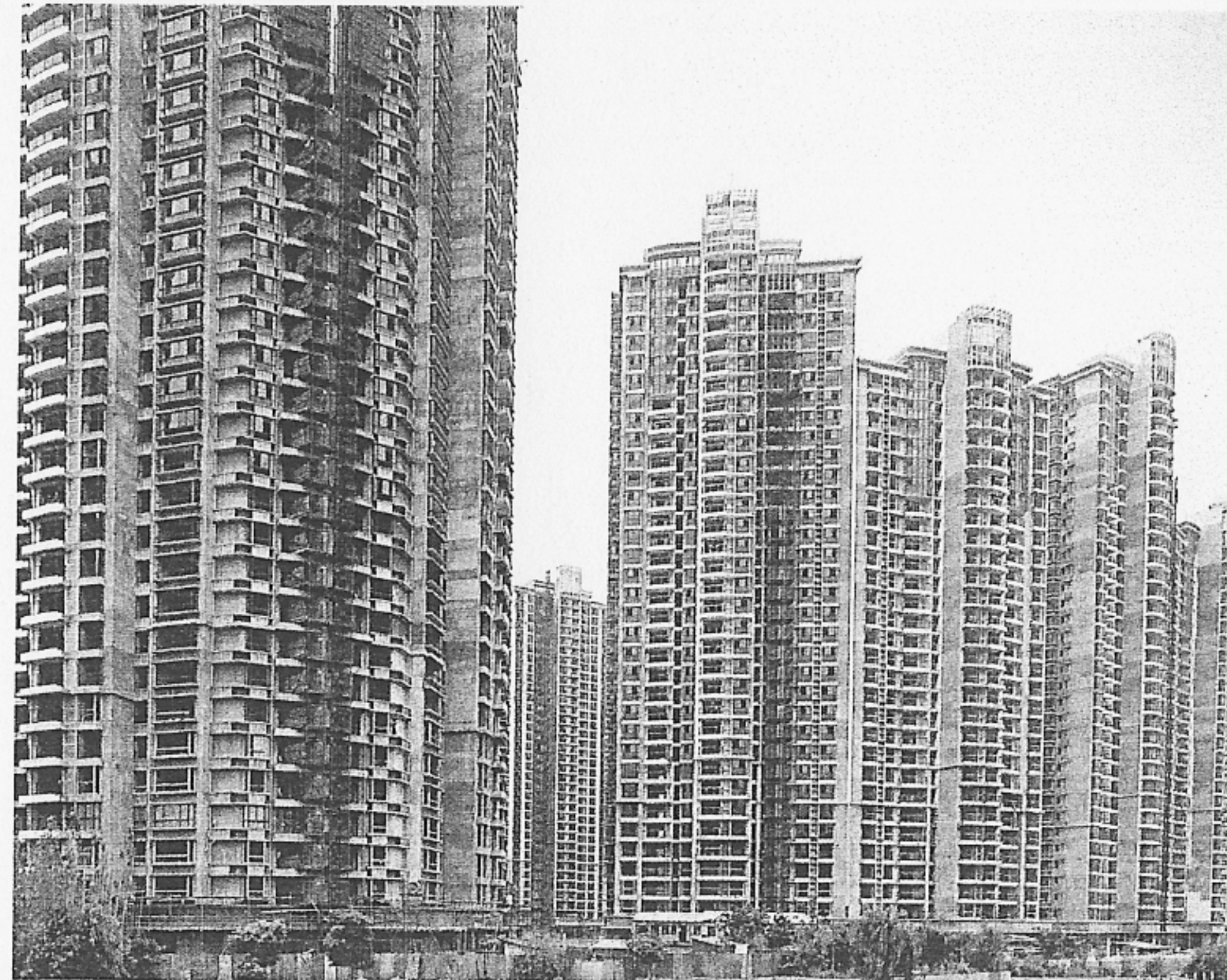
Left New residential towers being built north of Suzhou Creek
