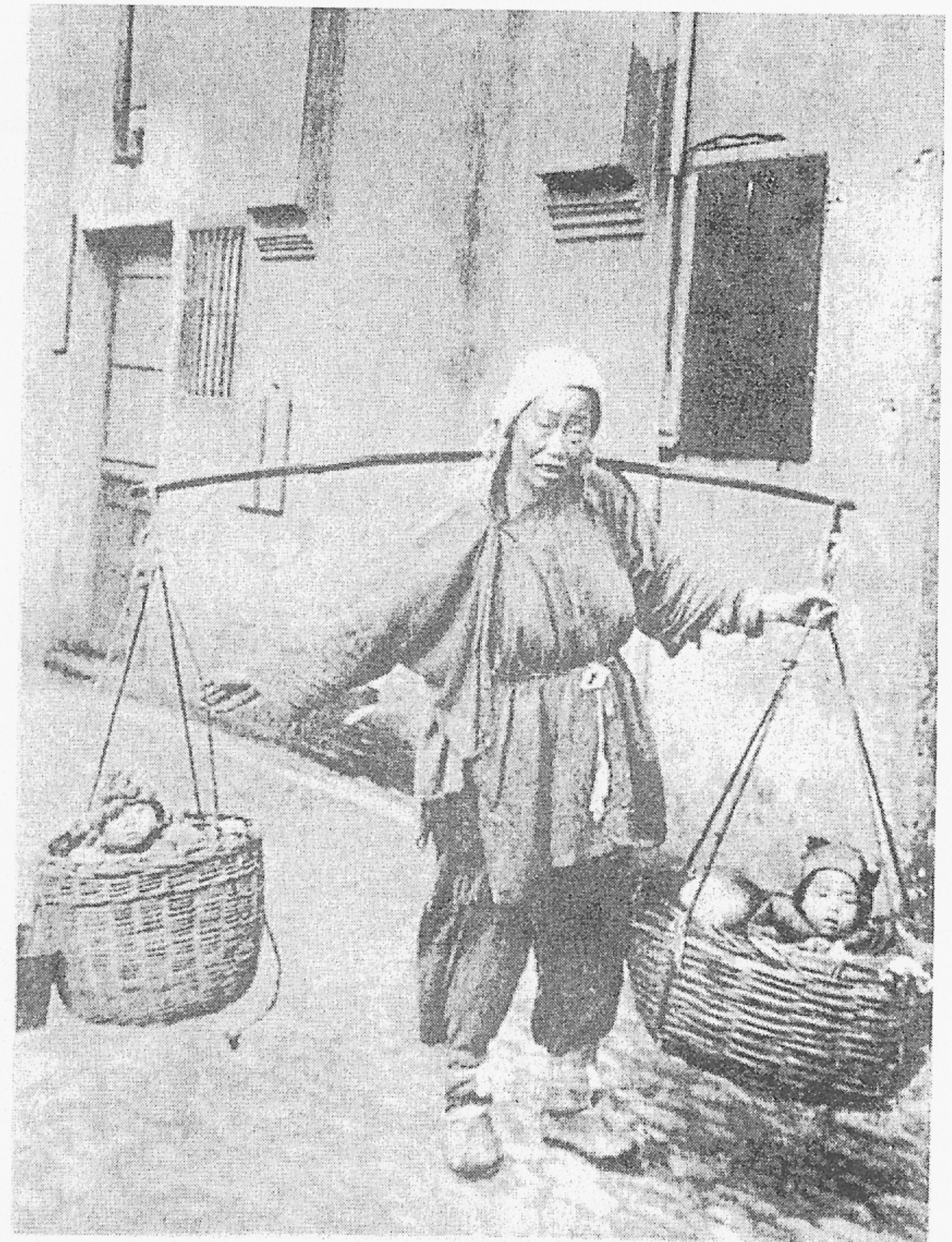
Fig. 3. In an alleyway, a newly arrived country woman carries her children and belongings in two rattan baskets. Immigrants like this often ended up living in a squatters' area but made a living in the city's better-off alleyway-house neighborhoods, working as domestic servants, street hawkers, tinkers, itinerant artisans, or the like. From R. Barz, Shanghai: Sketches of Present-Day Shanghai .
