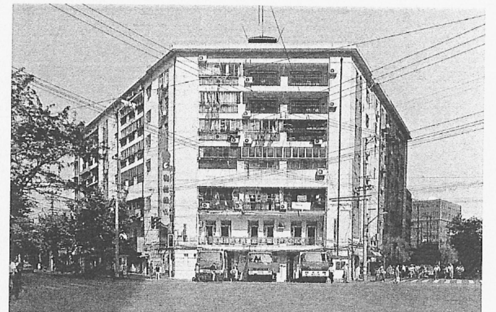
Above, left and right The three-storey fire station (C5) built in the 1930s near the former Bubbling Well (old) and in 2005 with an extra four storeys. The building has sunk by over two feet.
