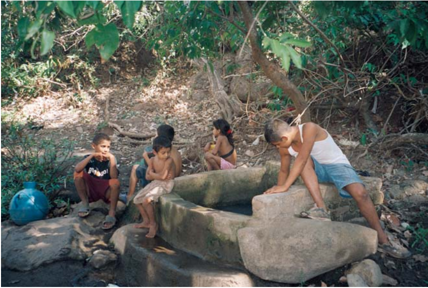
Date: July 5, 2009 Location: Porvenir Description: Springbox at river
